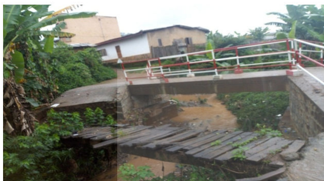
Figure 3: A newly constructed Bridge linking Cow Street and Ntarmulung
